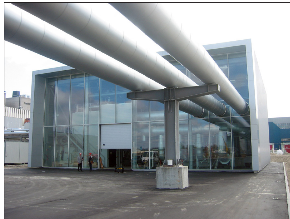
New pump building
